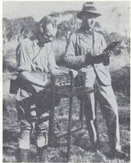
Figure 3. The Bieler Watson double detecting coil in use.
