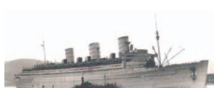
Fig. 15. 'Queen Mary' in 1940 showing the degaussing coil around the top of the hull installed in Sydney ( http://troopships.pier90.org/ships/q/queenmary ).
