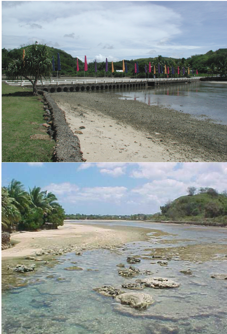
Figure 2. Top: Modern view of the resort causeway linking Yanuca Island with the mainland. Bottom: Yanuca Channel lagoon, downstream of the causeway at low tide, revealing dead corals and sand accumulation
