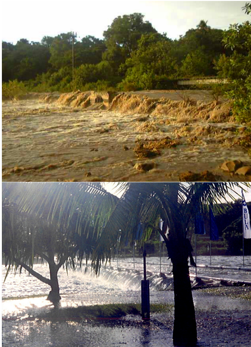
Figure 5. Top: Nalovo Creek in spate during an intense rainstorm on 4 February 2001; note the high turbidity of the water entering Yanuca Channel. Bottom: significant damming effect of the causeway in storm surge conditions during the passage of tropical cyclone Paula in March 2001. Source: Randy Thaman (USP) and the Fijian Resort.
