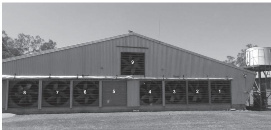
Fig. 1. Animal house showing ventilation fans at the end of the house.
