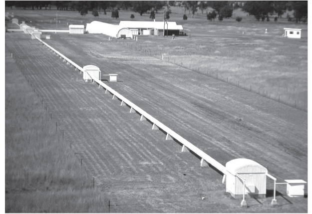
Figure 4 SUSI seen from the northern end of its 640 m north–south baseline array.
