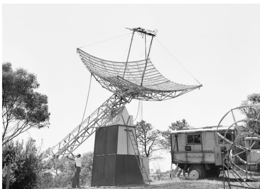
Figure 26 The 16-ft \times 18-ft paraboloid at Potts Hill field station in January 1952.
