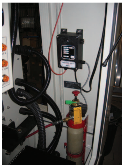
Fig. 8. The fire suppression control panel located in the right side of the electrical compartment.
