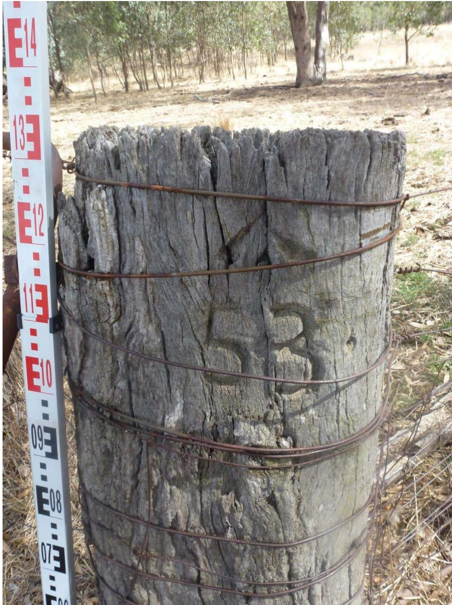
Fig. S8. A strainer post that has been marked by surveyors, situated on the corner of a Travelling Stock Reserve, Burrumbuttock NSW. Photo P. Spooner.
