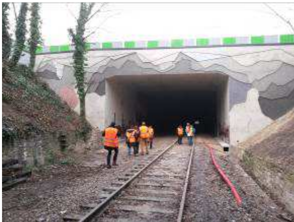
railway tunnel where the hibernaculum of pipistrelle bats is located
