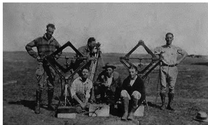
Figure 4. The non-contact receiving apparatus used by Elbof (from Elbof, 1927, p. 9).
