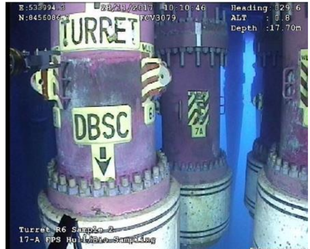
Lower turret and Diverless Base Stiffner Connections
