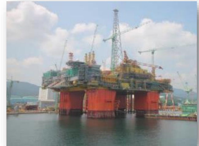
Ichthys Explorer - central processing facility (CPF)
