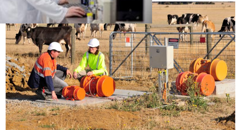
Testing Innovative Technologies
