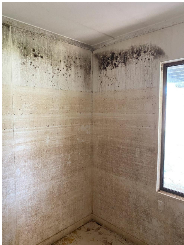
Fig. 1. Residential building wall mould growth above flood marked lines.
