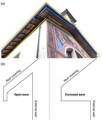
**Fig. 2.** (a) Photograph of building with open eave and exposed roof beams and enclosed eave, with soffit; photographed from below, and (b) schematic diagram of open eave and enclosed eave outline on a roof, eave, and external wall section.
